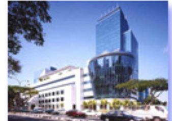
Police Cantonment Complex
